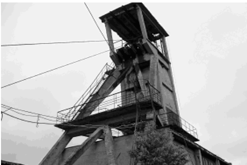
Fig. 3. The extracting installation „Puț auxiliar nr.2 ” Maleia Livezeni Mining Plant south- west view
