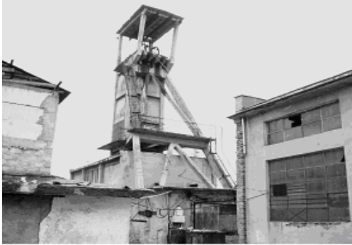
Fig.1. Extracting installation „Auxiliary well no.2“ Maleia Livezeni Mining Plant south – west view
