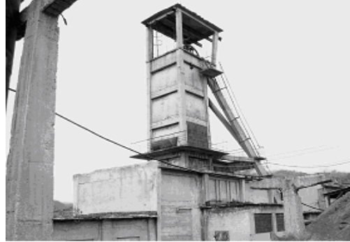
Fig.2. Extracting installation „Auxiliary well no.2 “ Maleia Livezeni Mining Plant north – west view
