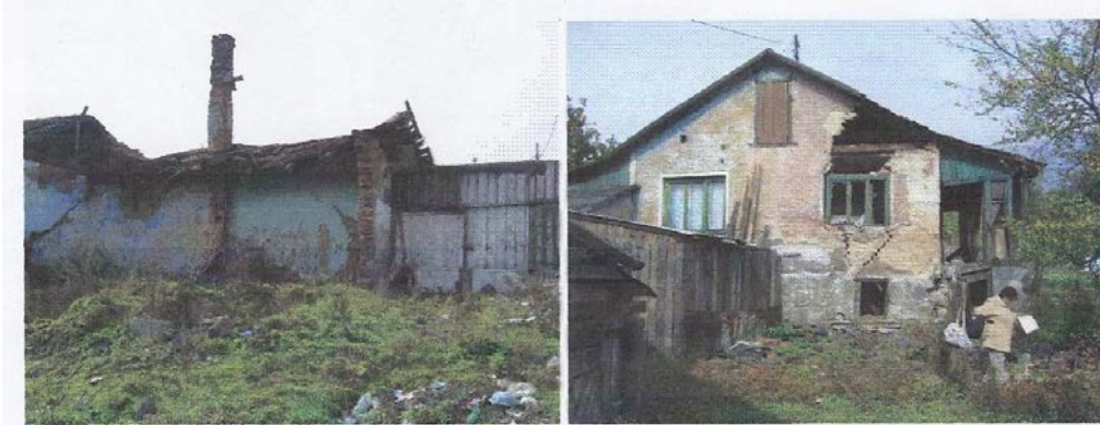
Figure 7. The influence of underground mining on some constructions, in the case of Lupeni Mine [2], [3]
